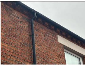
Photo of a site with the proposed works already carried out, which demonstrates increased depth of reveals and gaps to ground level.
